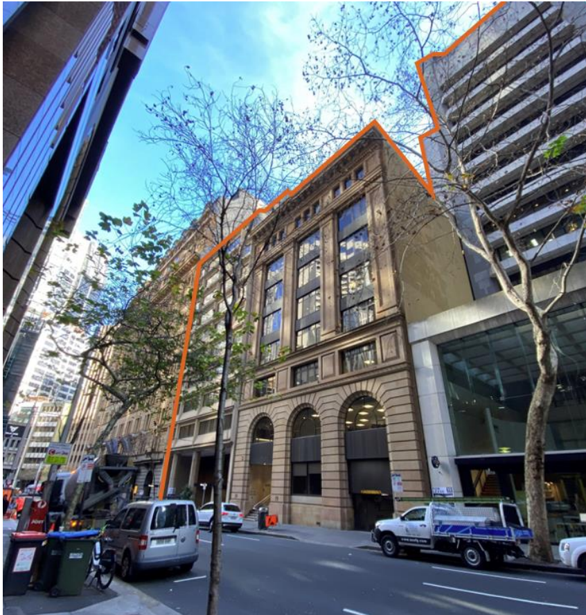
Figure 4: View from O'Connell Street, including the former Rofe Chambers heritage item at No. 19 O'Connell Street
