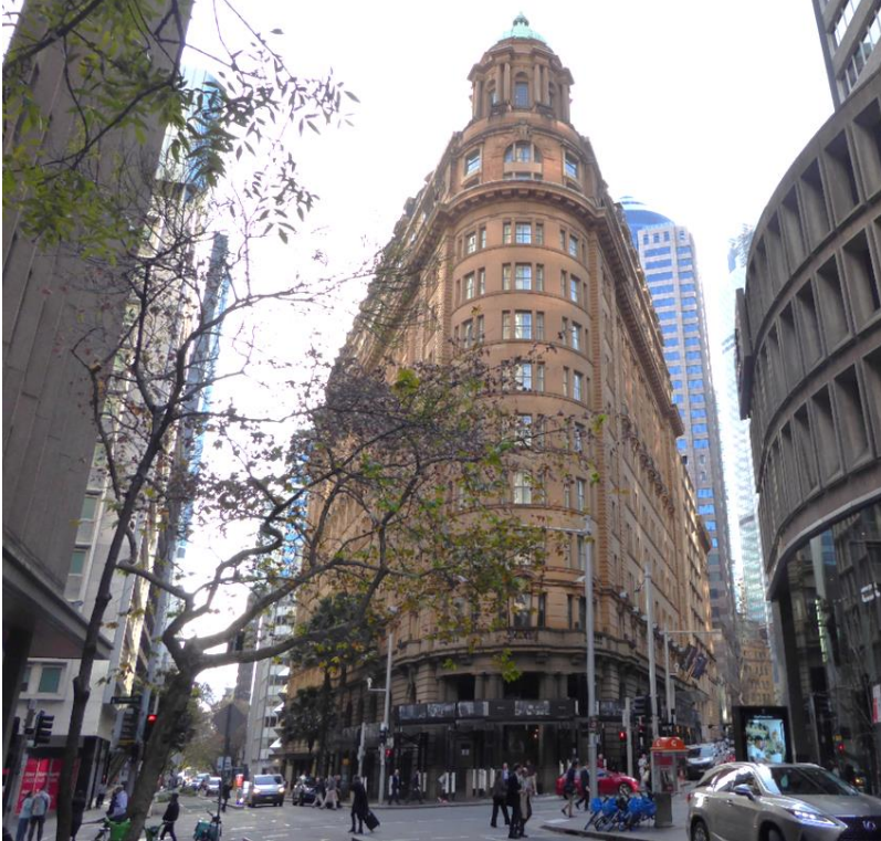
Figure 8: Radisson Blu Hotel building, with Pitt Street (left) and O'Connell Street (right)
